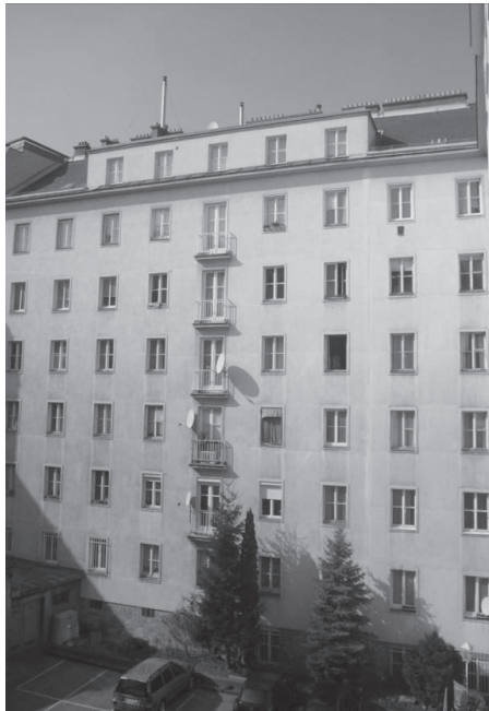
Figure 2: External View of Building B
