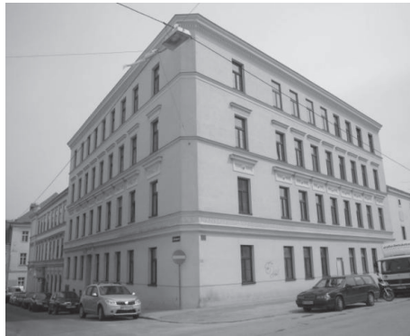
Figure 1: External View of Building A
