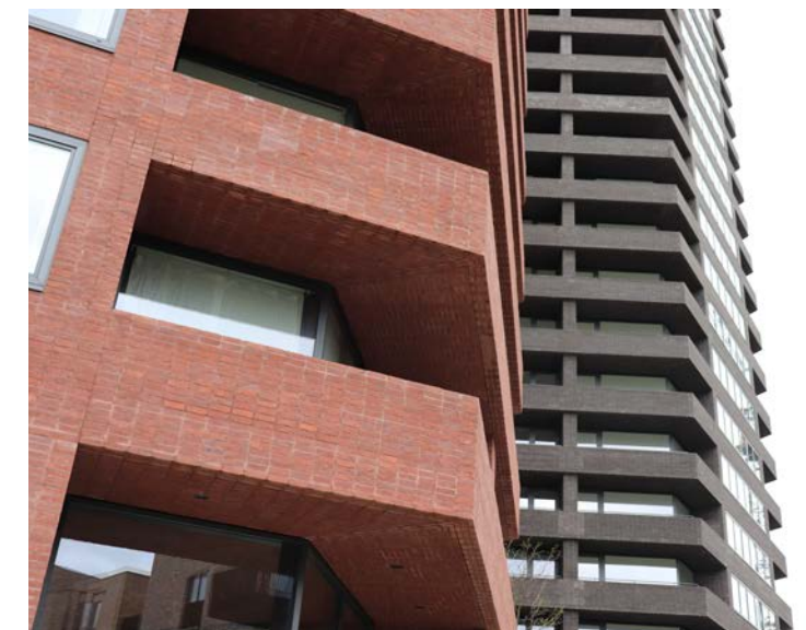
Colville Estate high rise residential
