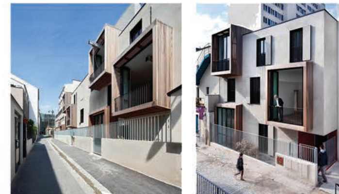
Above and below: Tetris social housing and artist studios frames the balconies , not only creating an interesting facade but adding a layer of privacy for inhabitants.
