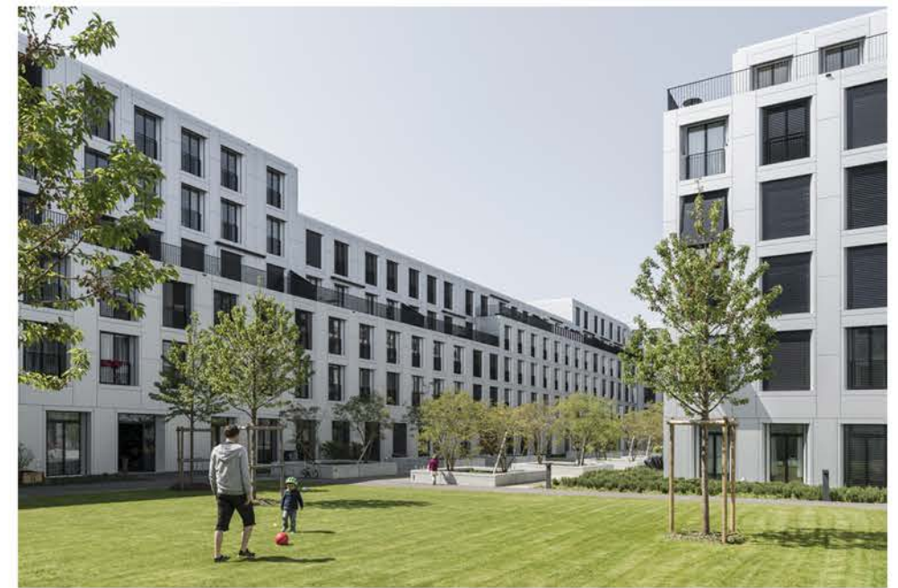
INTERNAL COURTYARD GARDEN
