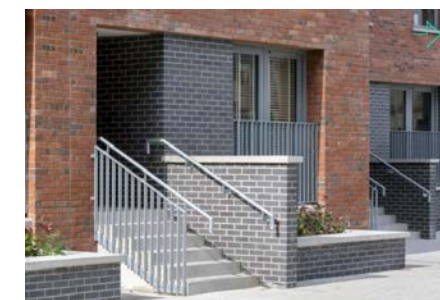
Liberty House, Dublin 1, Paul Keogh Architects
