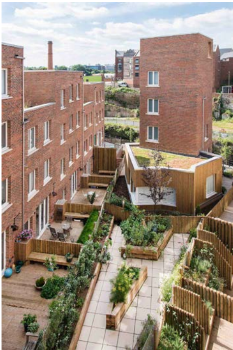
The Malings, Ouseburn, Newcastle by Ash Sakula Architects
