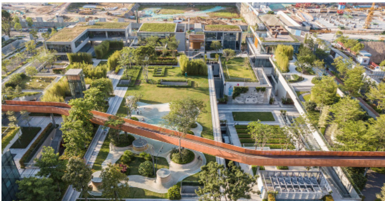
Vanke Design Community showing possibilities through roof gardens.
