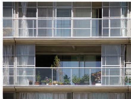
Above and left: Apartment renovation in Bordeaux by Lacaton & Vassal involved adding private winter gardens and external balconies to a post-war block
