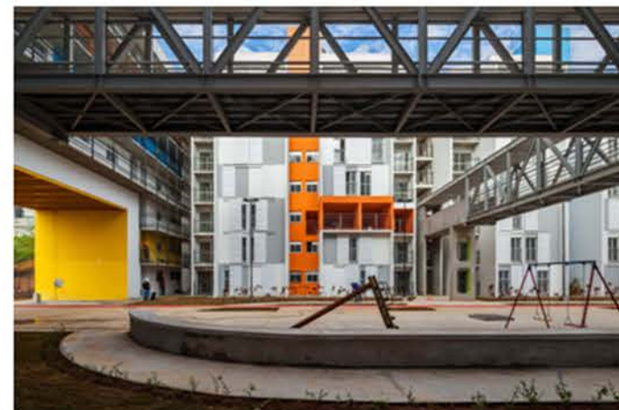
Left and below: apartment block in Grenoble by Édouard François with timber access routes pulled away from the building face to give privacy to inhabitants
