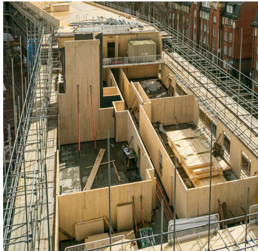
CLT Construction system in the block facing Rodney Road
