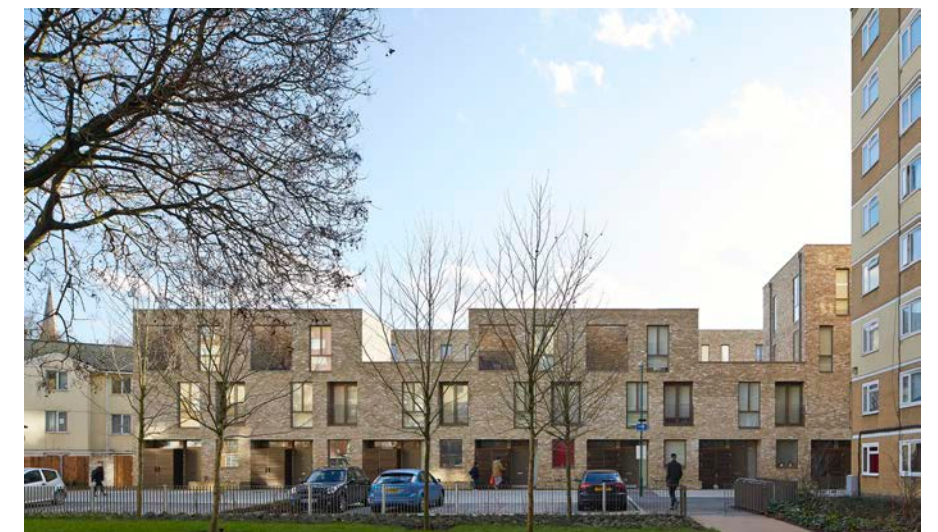
Mews building and connection to context, Alison Brooks Architects
