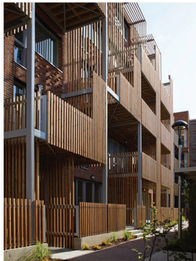
Below: Vertical timber slats provide shade and privacy for staggered balconies arranged across the facade of this east London housing development by architects Angela Brady and Robin Mallalieu
