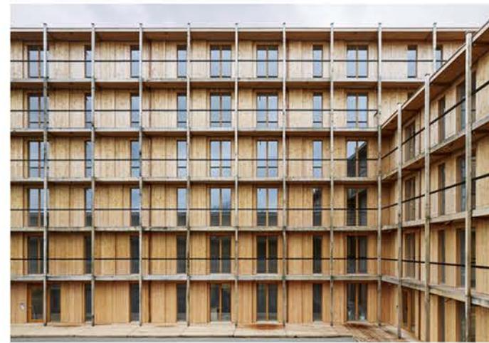
Left: Field 72 designed this block in Austria with shared deck access within an atrium Above: Hagmann Areal apartments in Switzerland is a small scale timber development with open decks and flexible spaces that can be adapted to suit the users needs.
