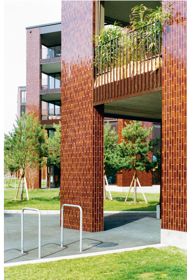
5.11 Ceramic tile facade, Katzenbach IV, 2020
